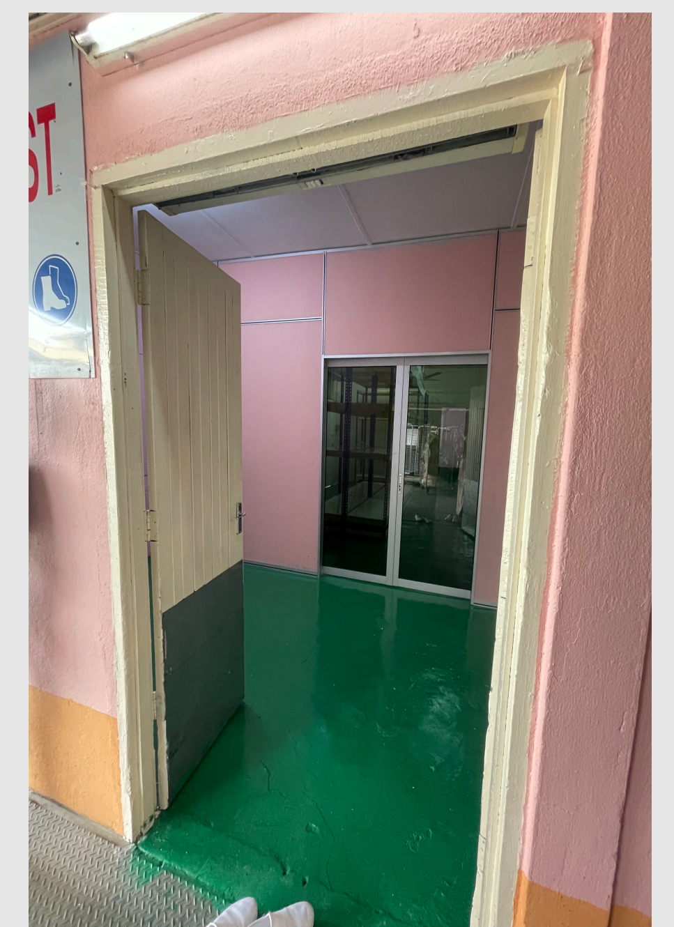
Figure 5. Linen store post renovation – anteroom
